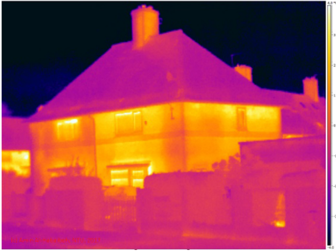
Fig. 1. An infrared image of a building in Nottingham UK.
