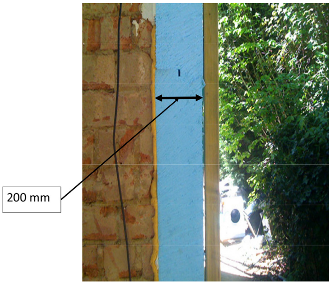
Fig. 7. A cross-section in one of the walls showing the external insulation.
