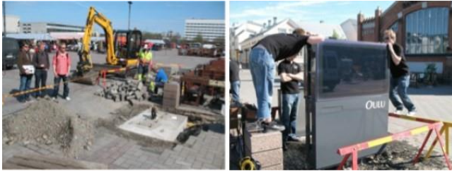
Figure 1. One of the Oulu displays being installed.
