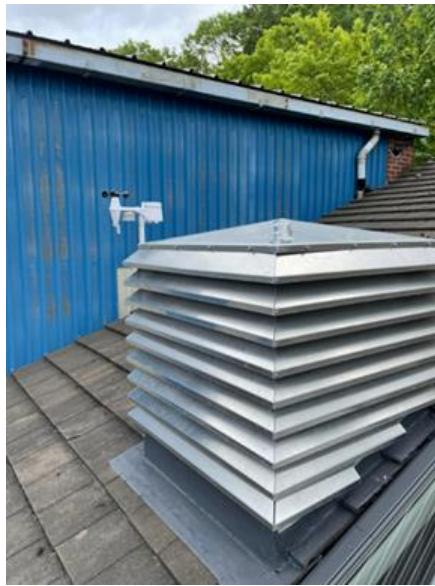
Figure 3 Wind tower installation
