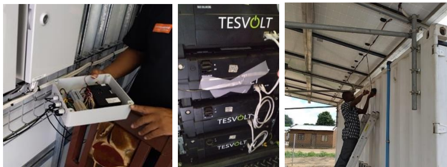
Figure 11 Logger installation in Malawi (left), temperature sensor on battery pack (centre), external air temperature sensor (right)
