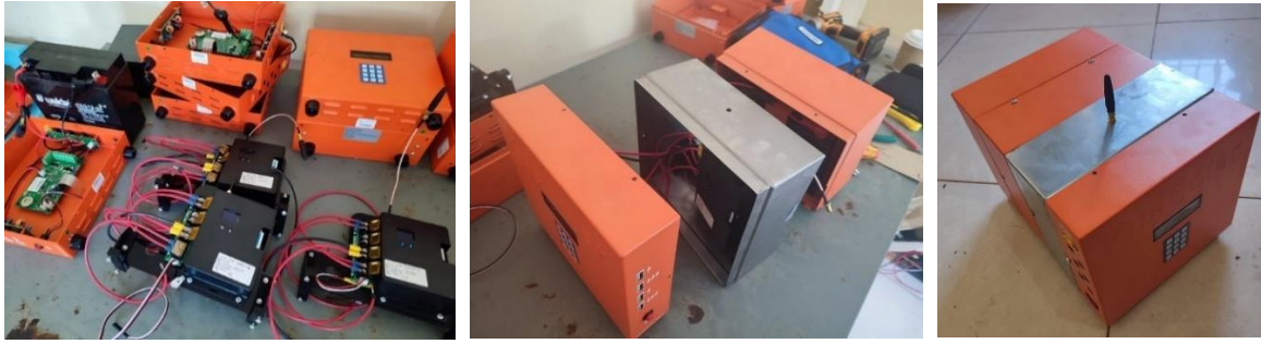
Figure 8 Installation of the logging equipment into the Kua SHS in Zambia
