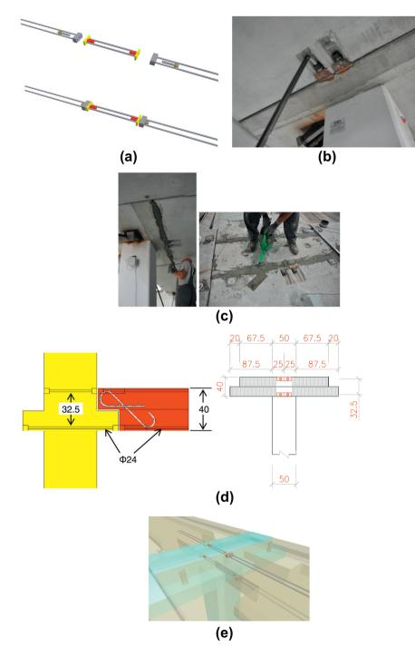
**Fig. 8.** (a) Loosen and activated connection system in its bare configuration. (b) Activation of the loosen bolts to provide continuity to the longitudinal bars crossing the beam–column joint. (c) Filling the gaps in the joints with mortar. (d) Detail of an emulative beam–column joint. (e) Three-dimensional representation of the mechanical connector in a central beam–column joint.
