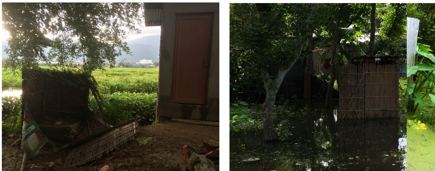
Figure 3: A pukka latrine built on raised ground to replace a dysfunctional phase 2 TSC latrine (left) and two seasonally flooded TSC latrines (centre and right).
