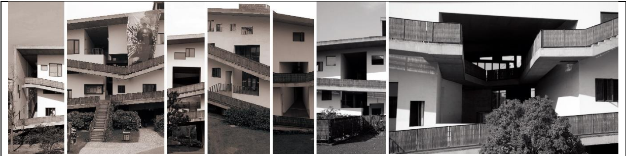
Figure 4. Several voids interrupting the horizontal extension of Building 18's space
