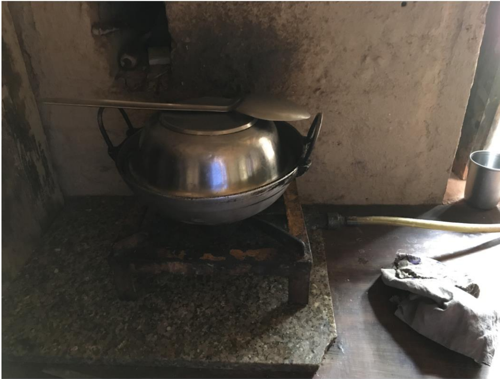
Figure 9. This biogas stove in Kavrepalanchok District, Nepal is fuelled by clean energy generated from household and animal waste. In addition to cooking gas, the biogas system produces digestate that can be used as fertiliser.
