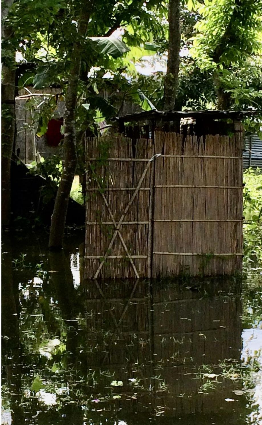
Figure 6. This toilet near Guwahati, northeastern India, gets flooded for 2–5 months per year. During this time, its owners have to defecate in the open or share their neighbour’s toilet which is built on higher ground. Open defecation is strongly associated with diarrhoeal disease which remains one of the most significant causes of ill health and disease in low income countries. Source: the authors.
