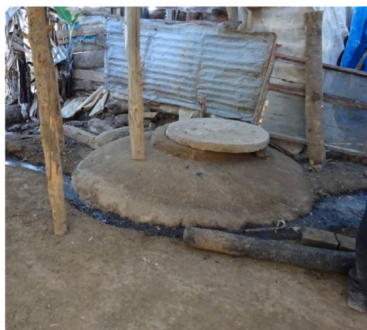
Fig. 1. Concrete fixed-dome biogas digester.
