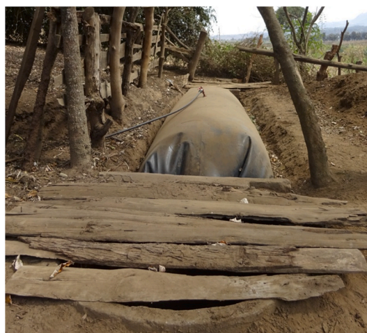
Fig. 2. Plastic bag biogas digester.
