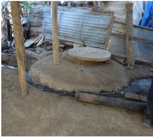
Figure 1: Concrete Fixed-Dome Biogas Digester
