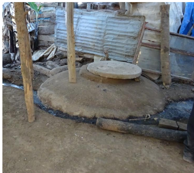
Figure 1: Concrete Fixed-Dome Biogas Digester
