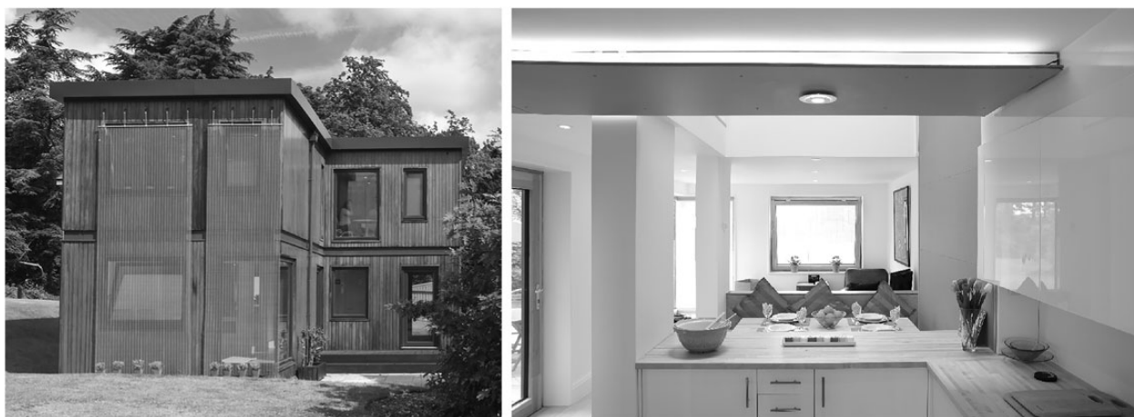
Figure 1. External view of the Nottingham HOUSE (left) and view of the interior (right) (Copyright The University of Nottingham).
