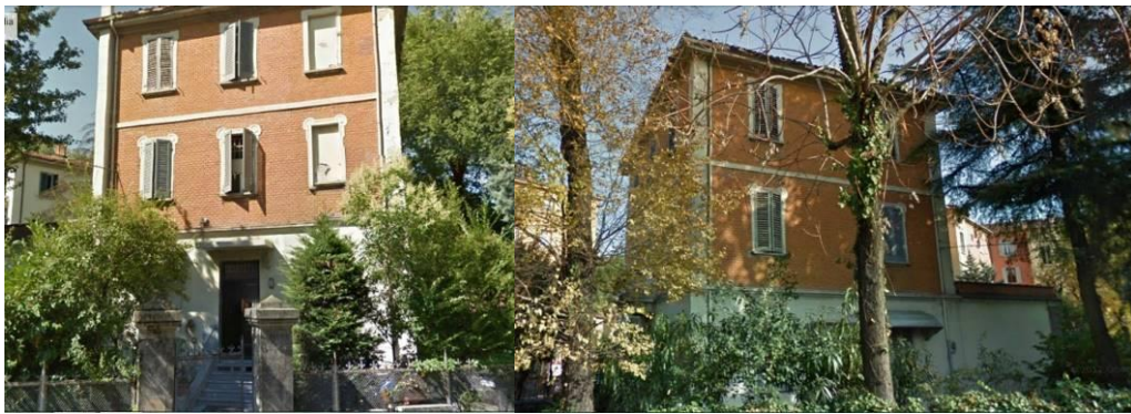
Figure 1: Street views of the house: Northeast side (left) and Southwest side (right)
