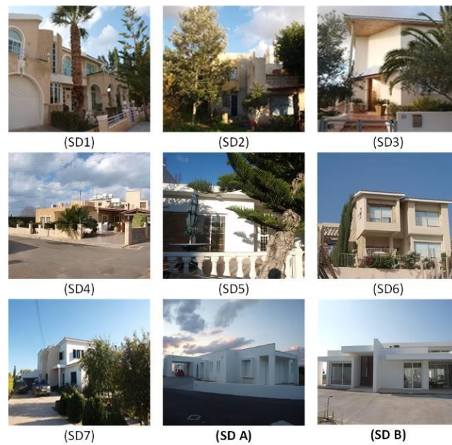
Figure 99 Exterior view of case studies
