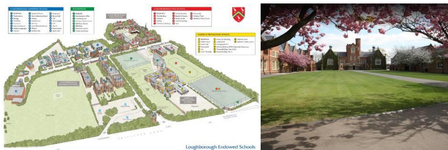
Figure 4: Typical historic Victorian brick building and building distribution in LES
