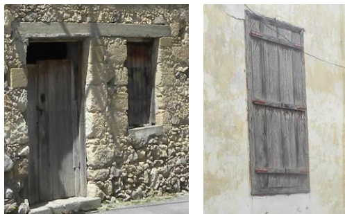
Figure 3: shading devices in Kozan and Bellapais Village
