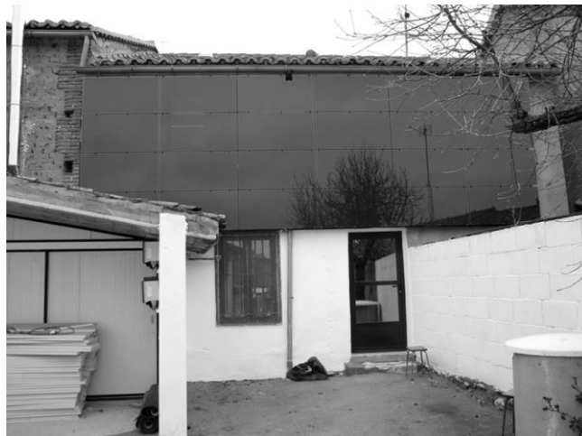
Figure 96: Photovoltaic ventilated facade of the Gotarrendura house
