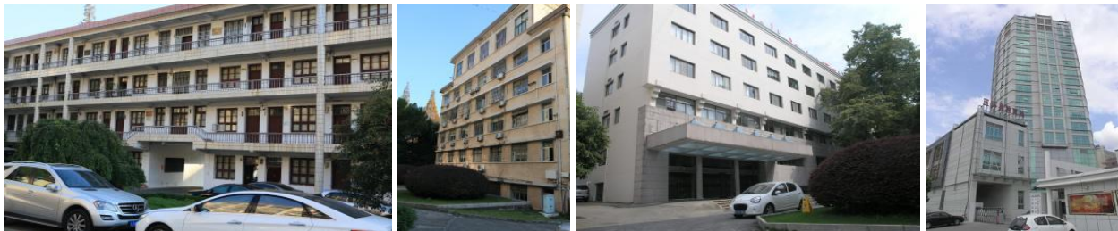
Figure 145: Office buildings A, B, C, D (from left to right)
