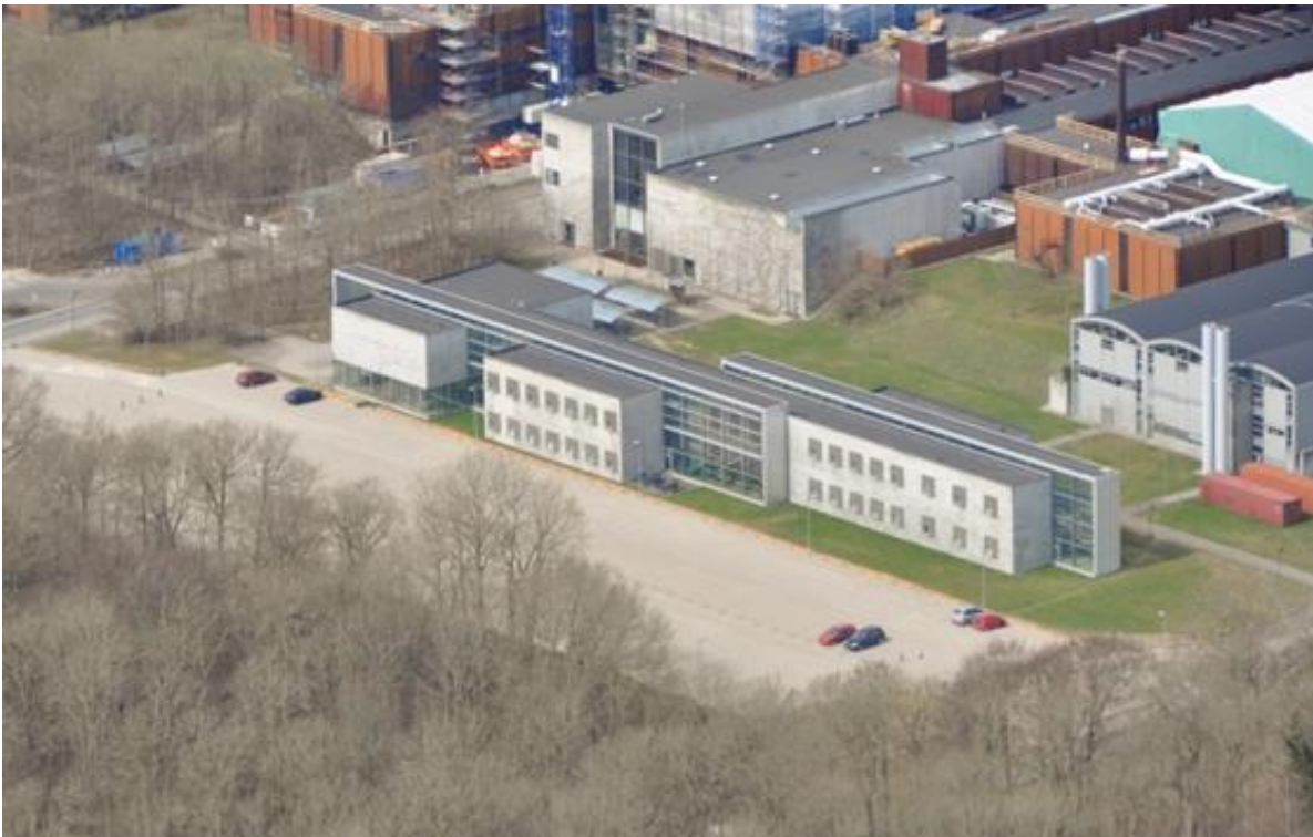
Figure 3: Maersk Office Building
