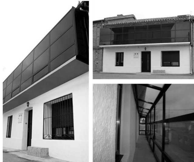
Figure 95: Photovoltaic gallery of the Gotarrendura house
