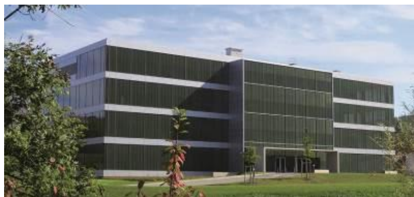
Figure 8: Pharma 2020, New building; Production Department; Sulzbach-Laufen, Germany. About 2000 m 2 aluminium structure with daylight redirection of the RETROLuxTherm 20 mm type, in insulation glass in combination with a glazing 50/25; ideal for large-area façades
