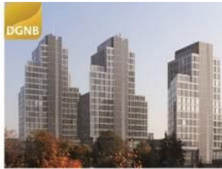
Figure 5: Litex/Sopharma Triple Towers, Office buildings, Sofia, Bulgaria. Non-ventilated double-skin façade with Fresnel blinds of the RETROFlex 80 mm type, U value <math>< 1.1 \text{ W/m}^2\text{K}</math>, g-value ~ 0.05 - 1 in case of high summer sun and open blind.
