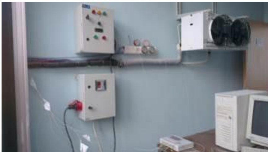
Figure 1. Indoor unit of air to air heat pump
