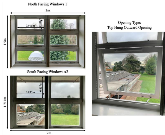
Figure 5. Marmont building lecture room window types.
