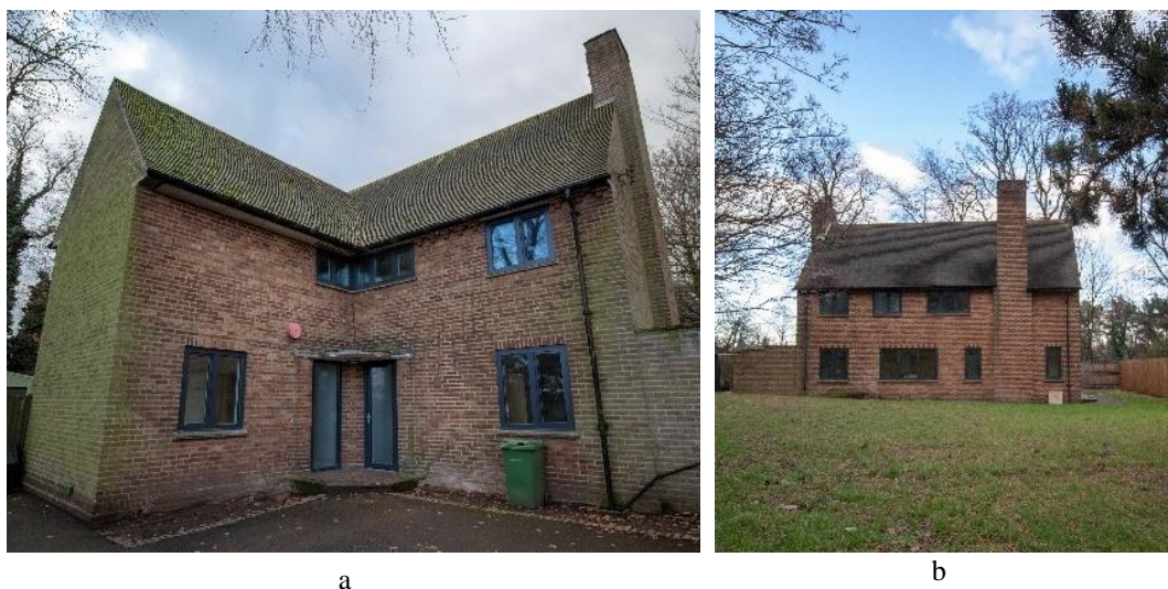
Figure 5: Tested building (a) front view and (b) back view
