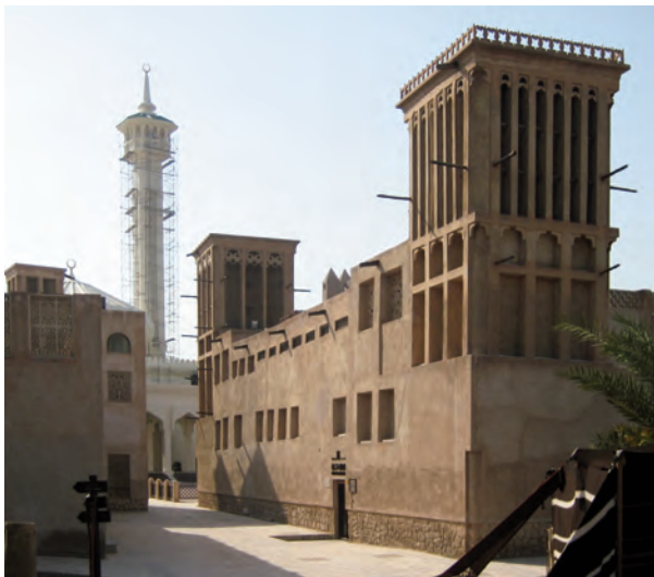
Figure 1. The reconstructed Bastakiya district in Dubai. (Source: Authors).
