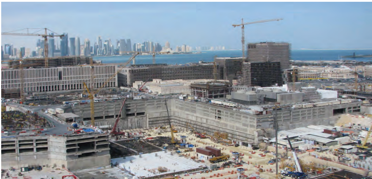
Figure 6. The Msheireb building site in 2013. (Source: Msheireb, 2013).
