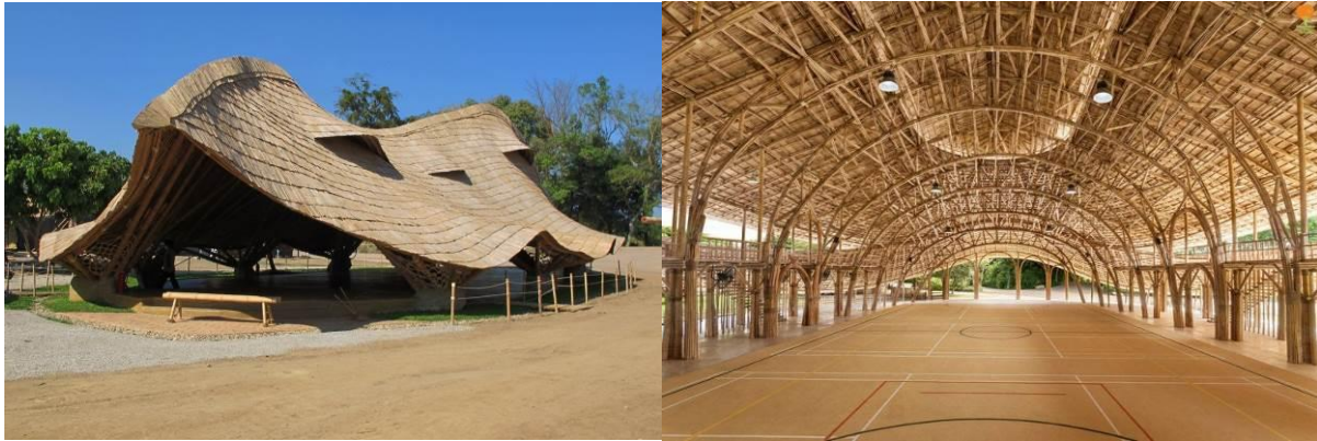
Figure 3: Panyaden International School Hall – 1 st hall damaged by flood in 2017 (left) and gymnasium hall (right) Sources: Left – the Author, 24 April 2016; Right - Chiangmai Life Construction (2012)
