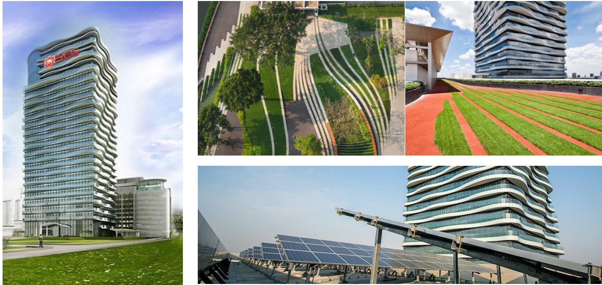
Figure 4: SCG 100 th Year building (left), landscape design for healthy lifestyle (top right) and solar roof top (bottom right) Sources: TK-Studio (2013).
