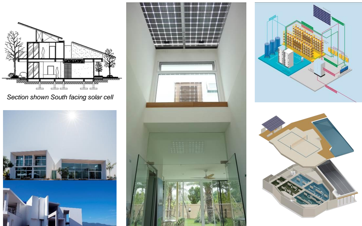
Figure 5: Phi-Suea House's orientation design (left), Phi-Suea House with solar roof (middle), Phi-Suea House's Hydrogen battery system (top right) and the underground cooling water system for Hydrogen energy management process (bottom right)
