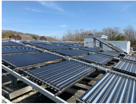
Figure 33: Evacuated tube solar collectors and cross-section of evacuated tube (Yamaguchi et al., 2006)
