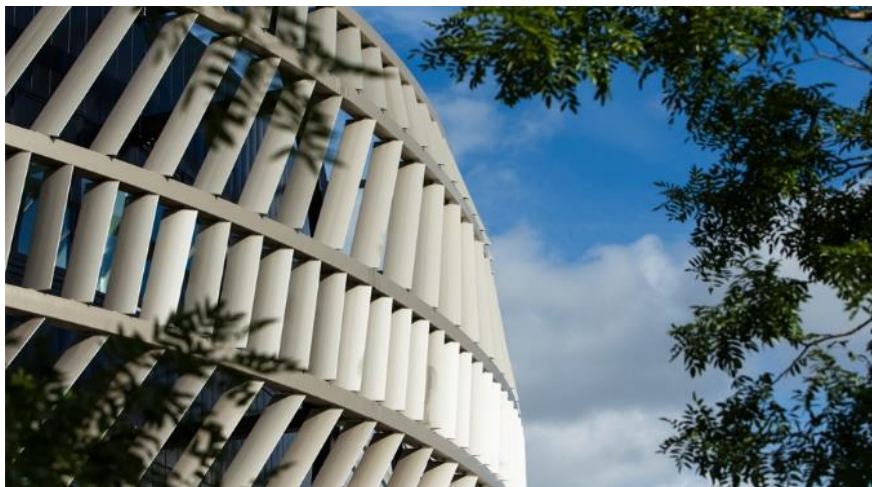
Figure 73: Shading devices of Ingenuity building (source: author)
