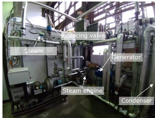
Figure 4: The main components of the steam-condensate circuit
