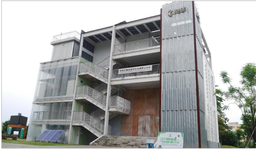
Figure 1: Practical building with PV and battery energy storage system
