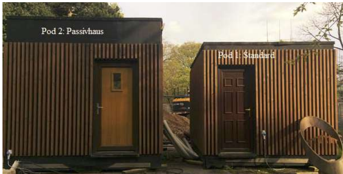
Figure 3 Test pods (left: a Passivhaus pod (pod 2), right: a standard pod (pod 1))
