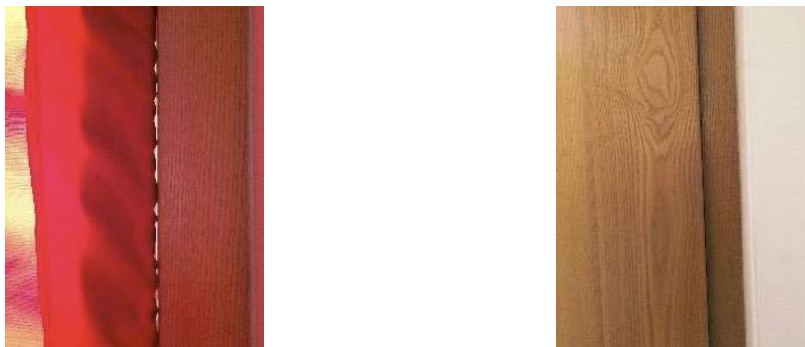
Figure 6 Difference between blower door installation (left) and actual door(right)
