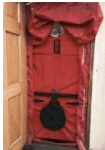
Figure 7 Setup of blower door
