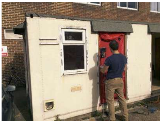
Figure 10 Setup of blower door (SW test)
