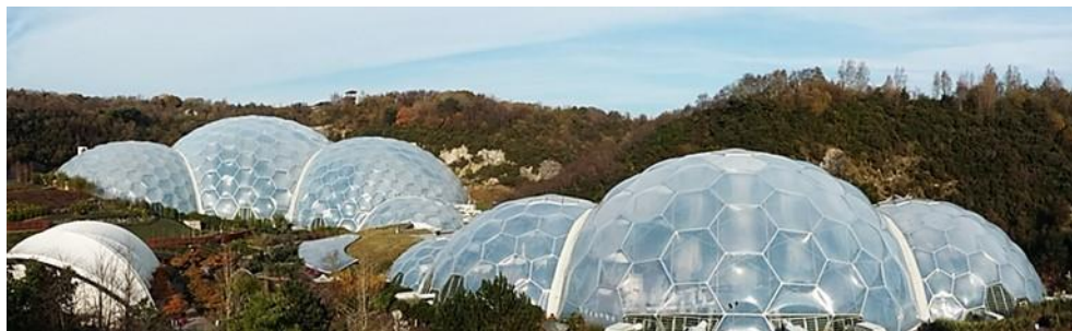
Fig. 1. Eden Project, St. Austell, United Kingdom (2000).
