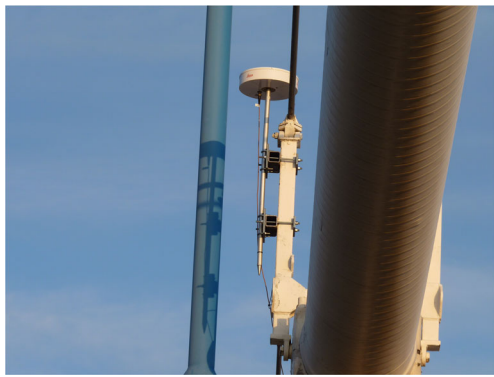
Fig. 7 Antenna located on the suspension cable
