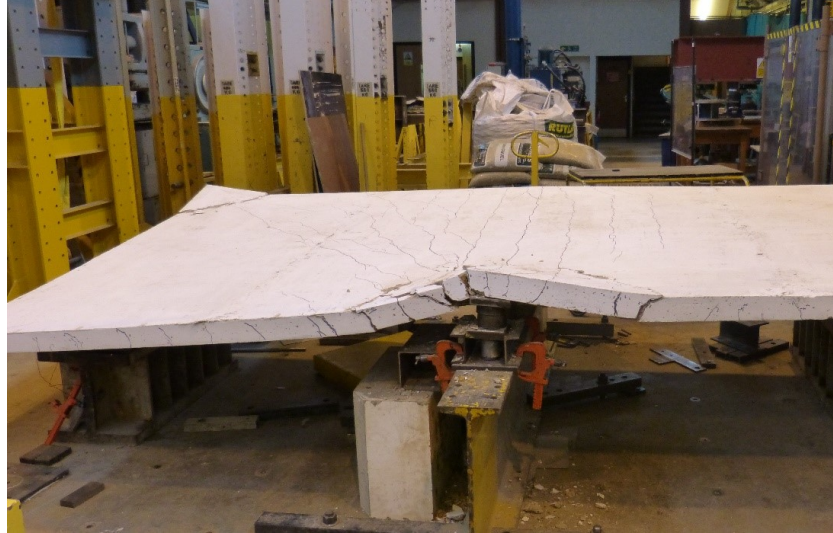
Figure 13: Final state of corner removal case after shear failure - Test C-D
