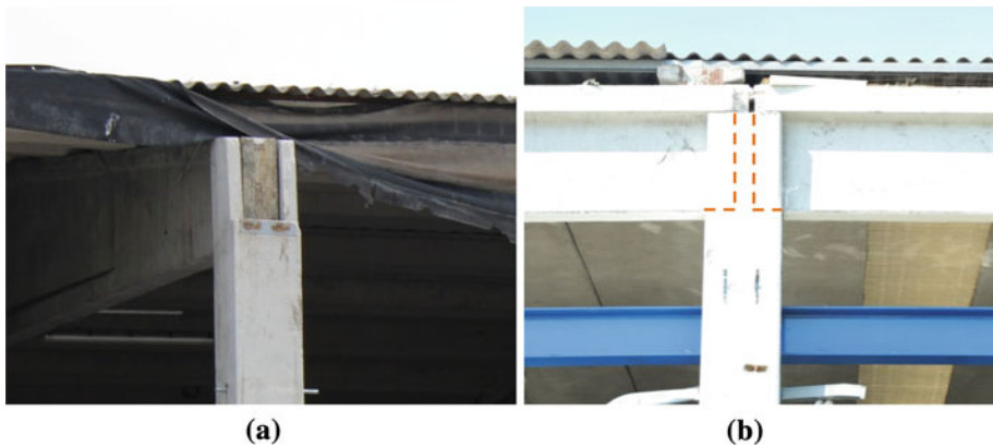
Fig. 7 a Seating of double slope precast beams showing the fork at the top of the column : seating at an end column . b Seating at an intermediate column of a “T” section beam (with dashed lines indicating the section of the beam at the seat pocket)
