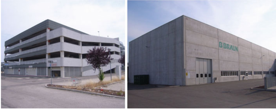
Fig. 13 Recently constructed precast concrete buildings exhibiting good performance
