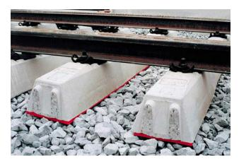
Fig. 1 Ballasted track with under sleeper pads
