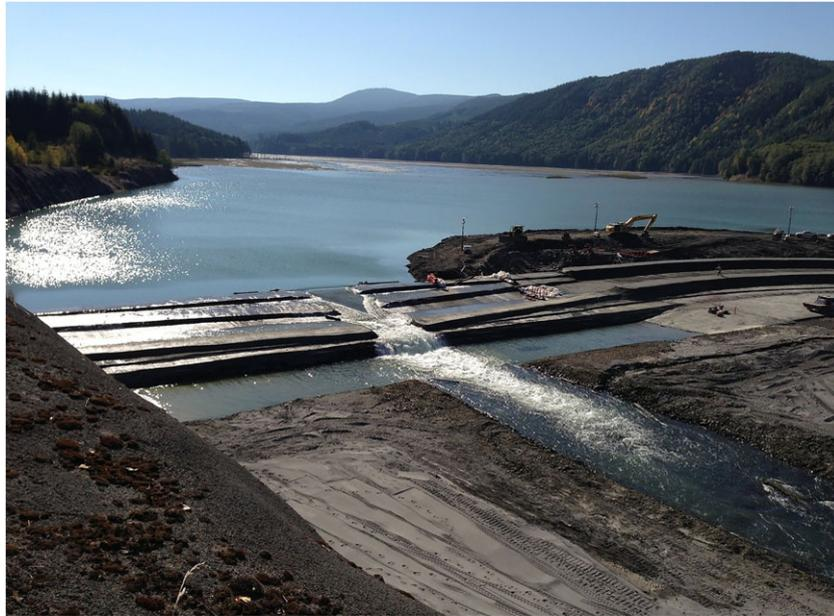
**Figure 8.** Pilot raise of the Sediment Retention Structure (SRS) spillway under construction during summer 2012. [Colour figure can be viewed at [wileyonlinelibrary.com](http://wileyonlinelibrary.com)]
