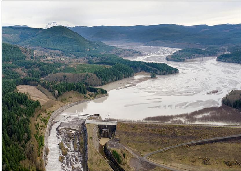
**Figure 3.** Sediment Retention Structure (SRS) and sediment plain in winter 2012–2013 (following implementation of the first spillway raise, in summer, 2012) (courtesy of USGS Cascades Volcano Observatory). [Colour figure can be viewed at [wileyonlinelibrary.com](http://wileyonlinelibrary.com)]
