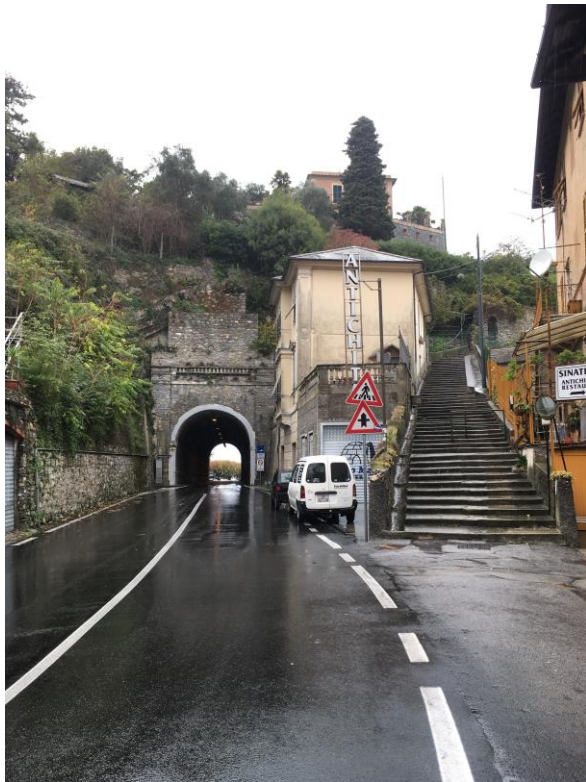
Figure 4. The Ruta tunnel, Charles Watkins, November 2017.
