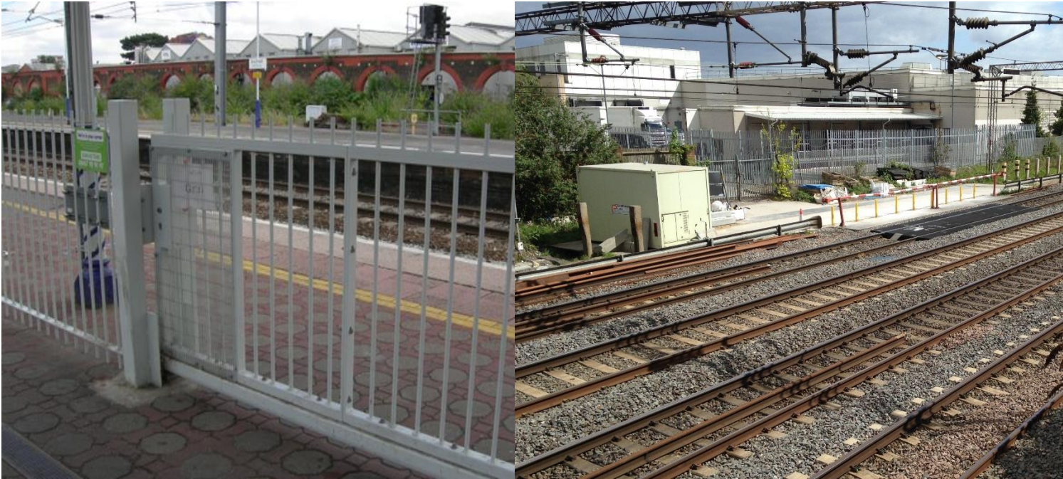
Figures 2a and 2b Photographs showing where a platform serving a fast line has been fenced off in an earlier intervention and where faster lines do not run close to platforms
