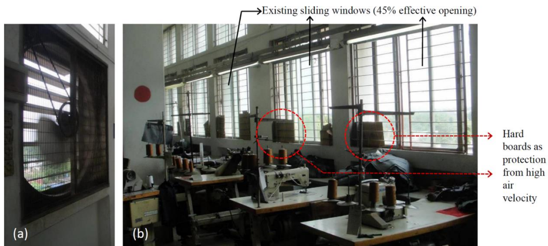
Figure 3. (a) Extract fans at ventilation outlets (b) Sliding windows at ventilation inlets with hardboard to protect workers from direct air flow
