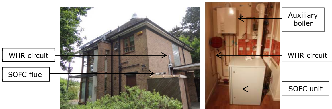
Figure 1 BlueGEN SOFC CHP system installed at The University of Nottingham
