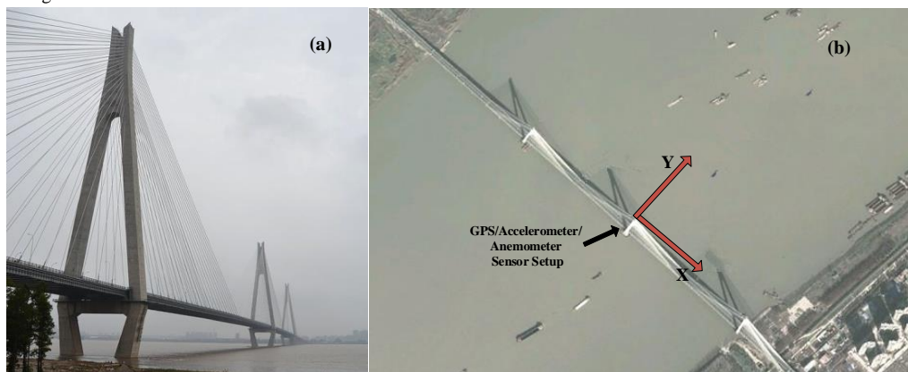
Fig.1.(a) The view of the Erqi Yangtze River Bridge in Wuhan ( http://en.wikipedia.org/wiki/Erqi_Yangtze_River_Bridge ) the local bridge coordinate system (BCS).
