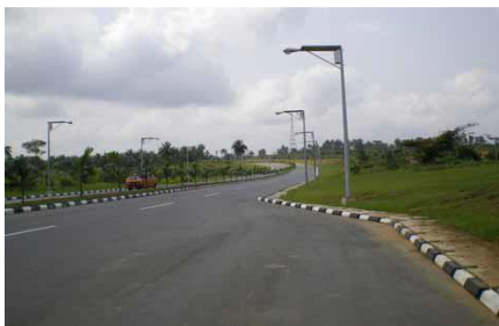
Figure 3: Solar Street Lighting in Uyo, Cross River State
