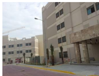
Figure 23 Chemical Department Building
