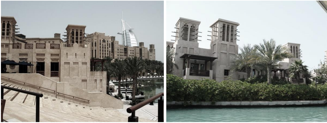
Figure 3 Illustrations of “non-functional” wind towers placed on top of buildings in Jumeirah, Dubai, UAE for aesthetic purposes [22].
