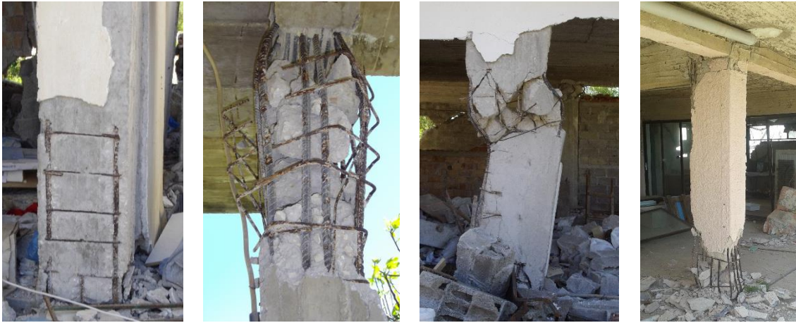
Fig. 1. Damage in RC columns due to old-type detailing (photos are taken by the authors).
