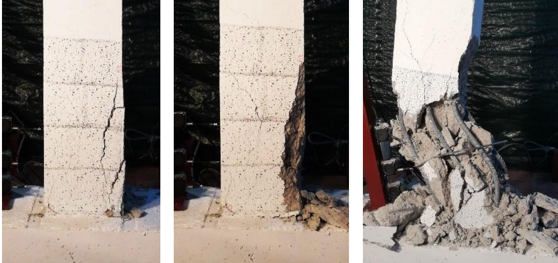
Fig. 8. Evolution of damage in the control cantilever.
