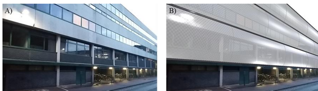
Figure 1: A) Picture of a south-east facing façade of an office building built in 1959, in Nottingham, UK. B) Artistic rendering showing a switchable ETFE double-skin façade added to the original building in A)
