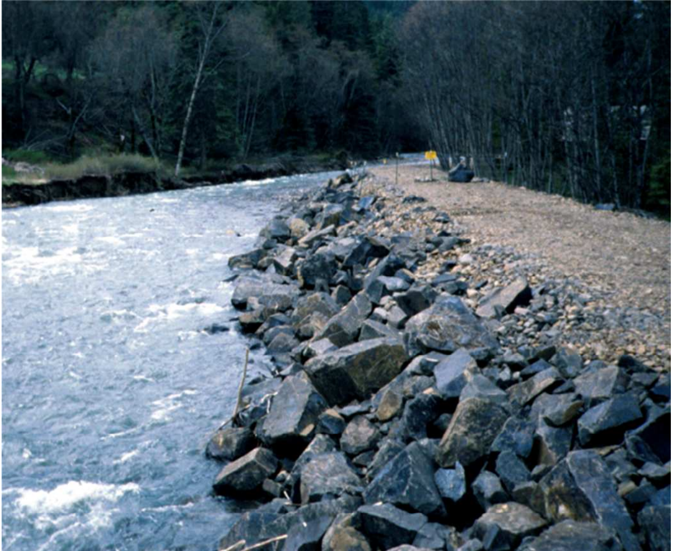
Figure 5. Riprap provides rigid bank protection that reduces the capacity of the channel to absorb the effects of short-term disturbances in the fluvial system and accommodate the impacts of long-term evolution.
