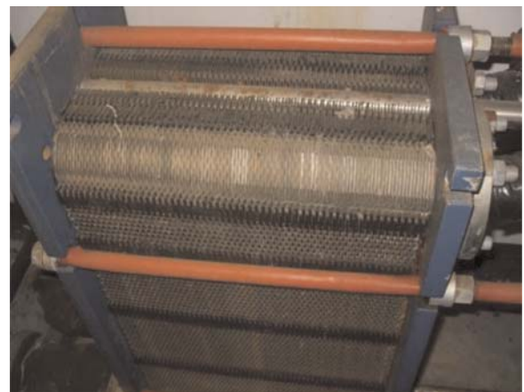
Figure 4. Flat-plate heat exchanger.
