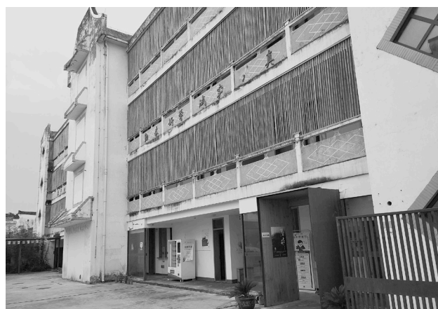
figure 15. An old primary school remodeled into a hotel in Xi Xi Nan. The classrooms were updated into hotel rooms, and a curtain of bamboo poles was added to the facade, which deteriorated after several years' usage. Photo by author.
