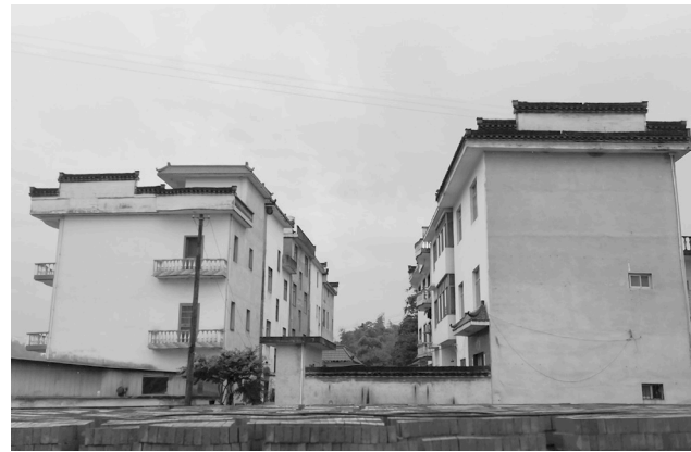
Figure 12. The nonsensical addition of matouqiang on the street side of buildings as the result of the gai hui policy. These buildings were not originally built in the Hui style. Photo by author.
