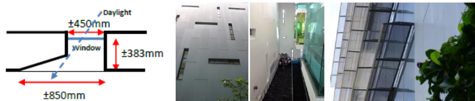
Figure 13: Left - Plan of Splay Angle Aperture. Source: Sketch by Author. Right - Splay Angle Recessed Window Apertures at East Façade. Perforated Horizontal Shading Device at South Façade. Source: All Photos by Author.
