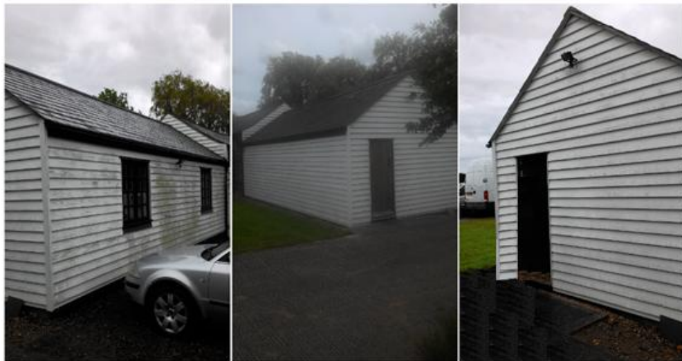
Figure 3: The test house which was integrated with the novel heat recovery system.
