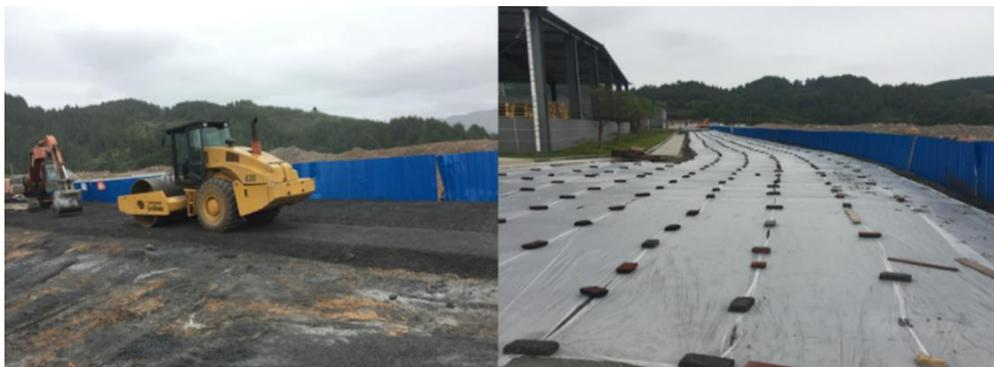
Figure 13. Field-test for road base material prepared with red mud [96]
