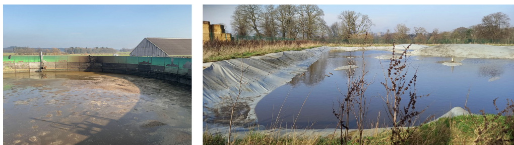
Figure 7. Slurry tank (left) and lagoon containing approximately 8 million litres of manure (right), UK dairy farm. Manure lagoon is covered by white geomembrane liner cover, with vents. Rainwater has accumulated over the canopy. Large upward bulges (whales) may be lifted up by underlying volumes of methane.
