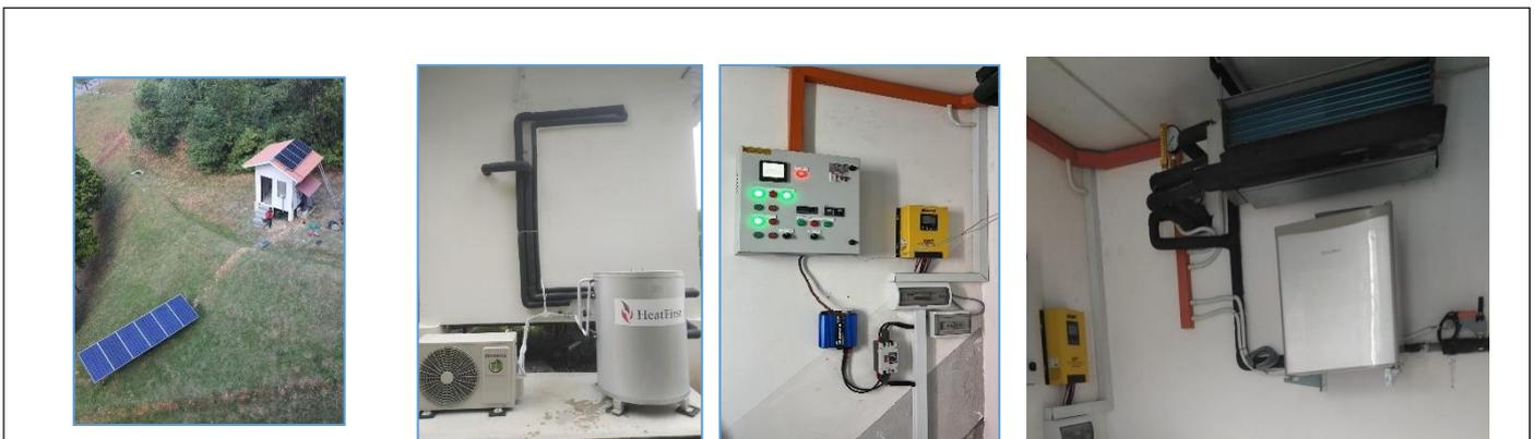
Figure 2: (a) The PV setup and the test house used for the case-study (b) The setup for the vapour compression unit and the thermal storage unit (c) The Balance of System (BOS) for auxiliary components and (d) The fan coil unit
