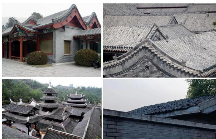
Figure 1: Integration of curved elements of traditional Chinese roofs
