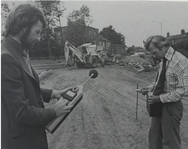
Figure 8: Image entitled "Noise reading being taken on a building site" from Noise Advisory Council, The Darlington Quiet Town Experiment: September 1976-September 1978 (London: Her Majesty's Stationary Office, 1981), p.15.
