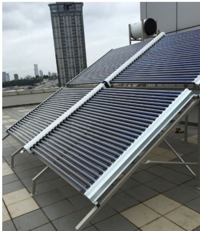
Figure 3: The schematic shows of the ETHP collector
