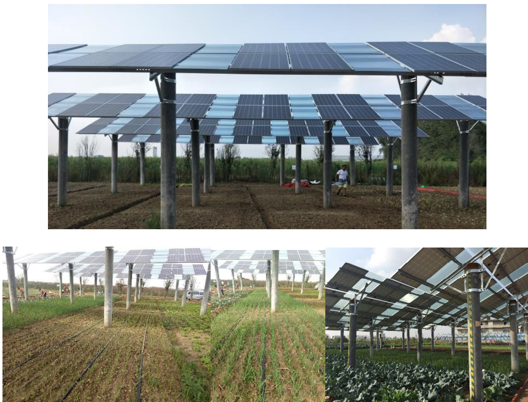
Figure 5: Photo of the Fuyang City TGPV project (Anhui Province)
