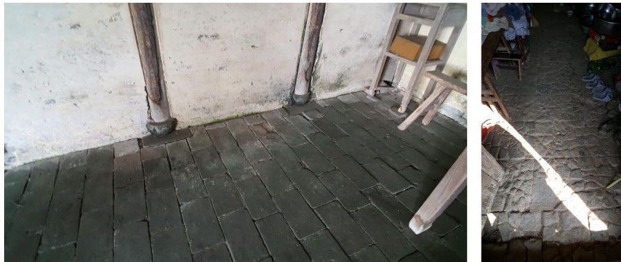
Figure 6: typical floor materials
