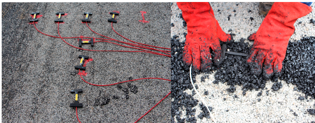
Figure 4. On-site installation of sensors in the pavement structure.
