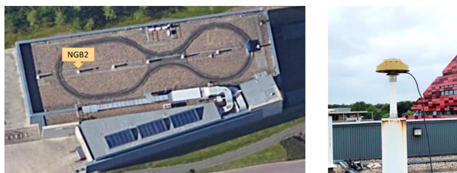
Figure 7. (Left) View of the roof of NGI building, with the location of control point NGB2 and (right) the GNSS antenna installed on the top of the pillar of NGB2.
