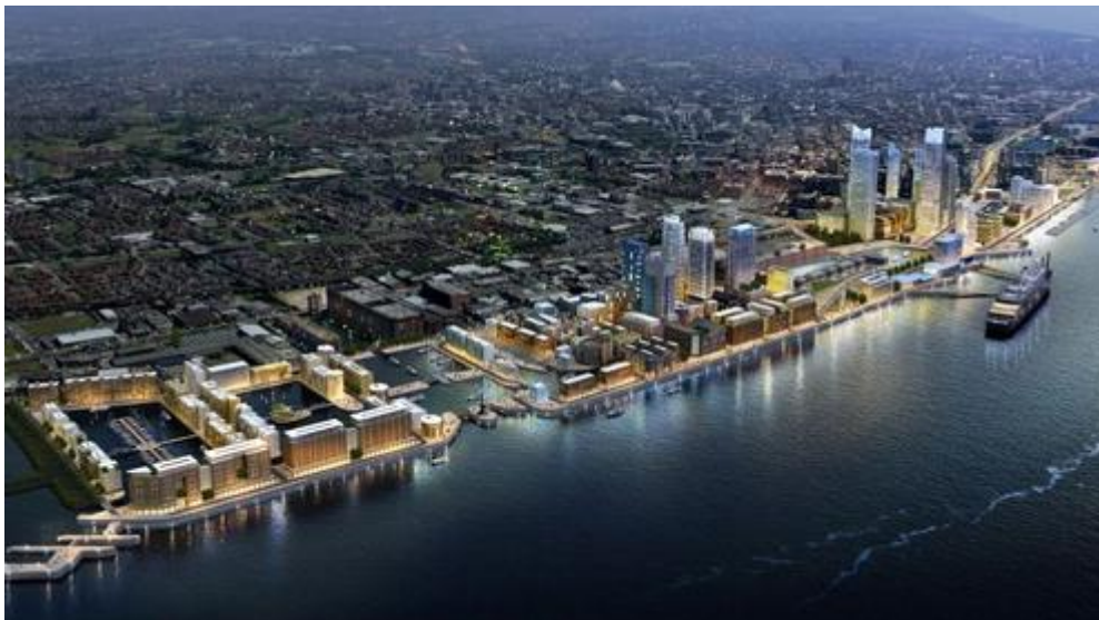
Figure 6. Computer Generated Image of Liverpool Waters project, the image shows the significance of the project and the two clusters of tall buildings which UNESCO is very critical about. Source: Chapman Taylor website (Liverpool Waters Project).
