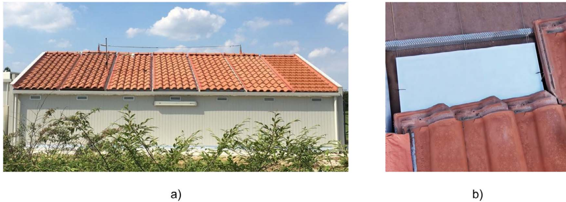
Figure 1. (a) Mock-up building at the TekneHub Laboratory at the University of Ferrara. (b) Arrangement of the PCM plastic containers in the ASV layer of the roof.
