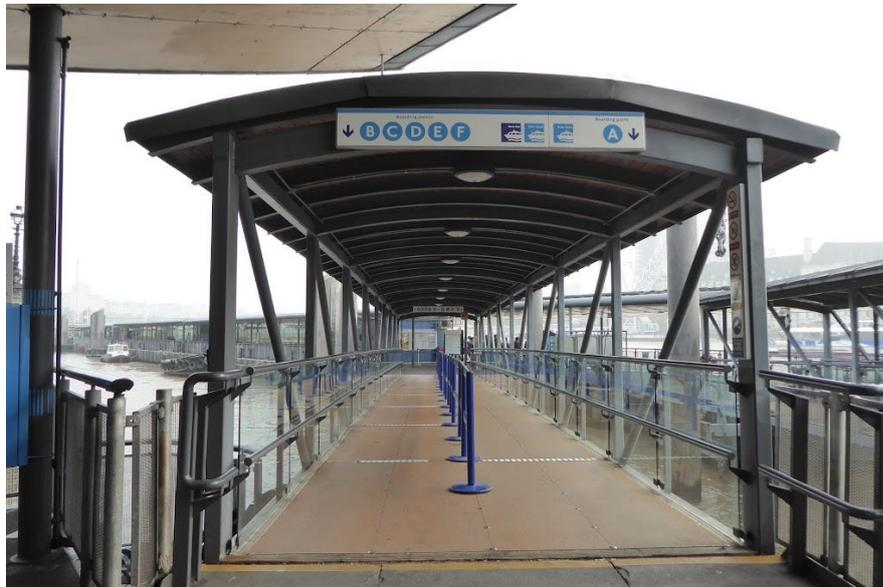
Fig. 1. Pedestrian truss bridge with CHS brace and RHS chord at Westminster Millennium Pier in London [3].
