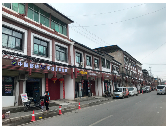
Figure 11. The current rural dwelling partly transformed into grocery stores and restaurants (i.e., China Mobile Limited, Noodles Restaurant shown in the figure) alongside the main street (source: the authors).
