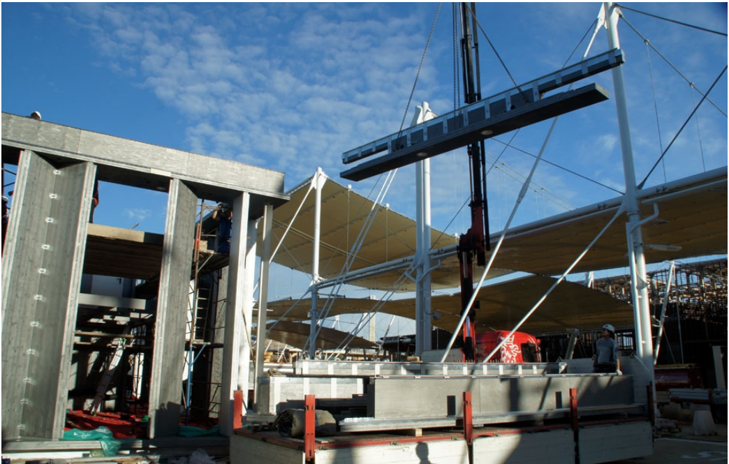
Figure 4: Assembly of the timber structure on site.
