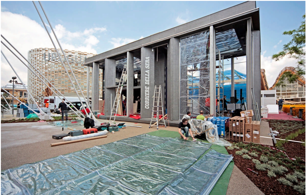
Figure 5: Assembly of the PVC envelope on site.
