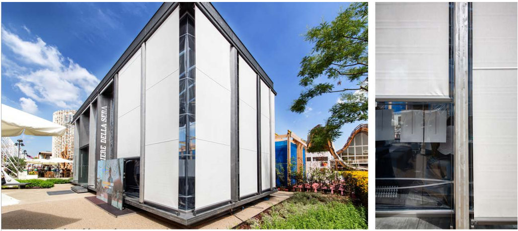
Figure 6: The external roll blinds (left) and the detail of the connection with the timber frame (right).
