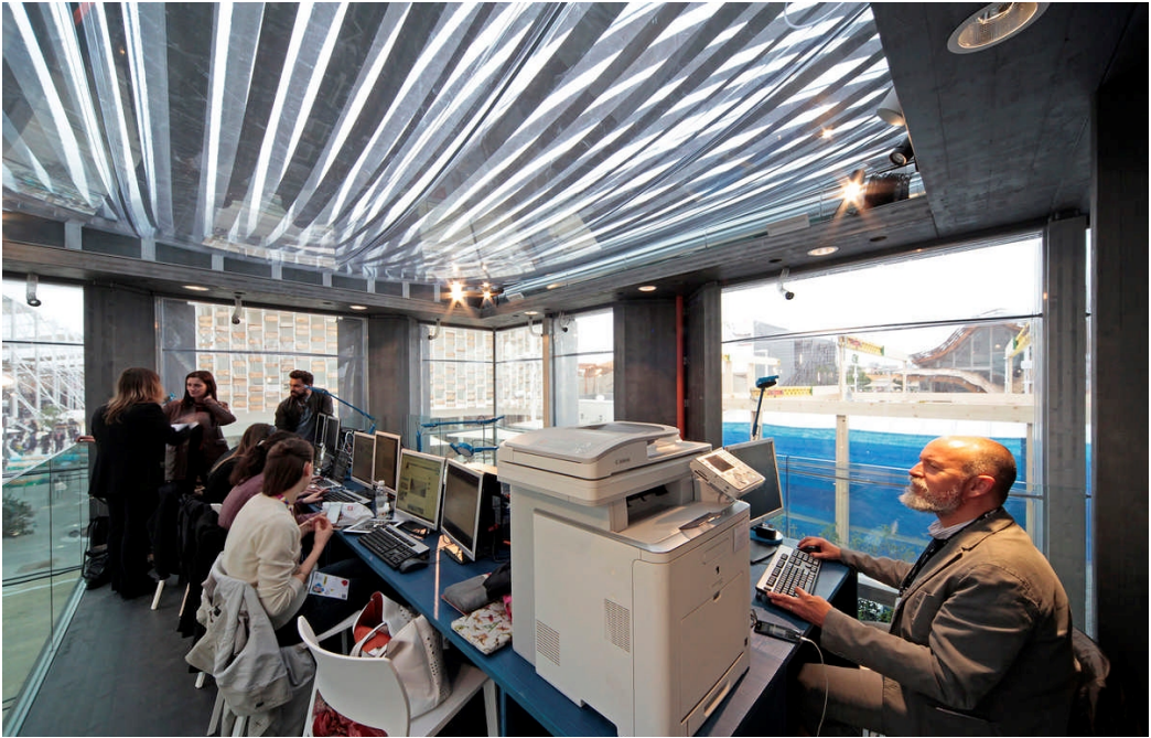
Figure 7: Detail of the two large skylights with the printed pattern designed to control the daylight.
